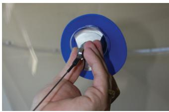
5. Install Fast-Fit™ alignment plate onto the retaining cable (or pipe) and into the bin with the shoulder positioned outward. Center the alignment plate in the mounting hole, aligning it in the vertical position with the arrow pointing upwards.
